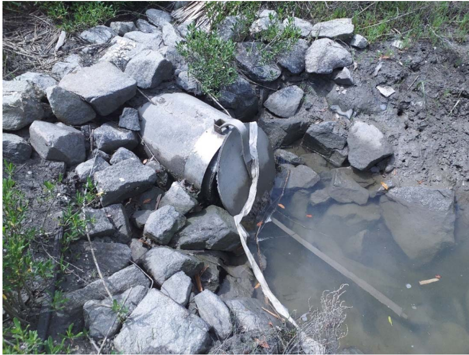
Exhibit B: The outfall Tide Gate currently is inoperable due to obstructions.
