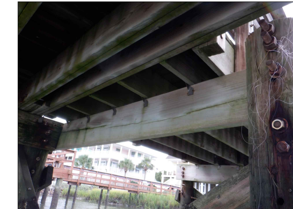
PHOTOGRAPH 2 - APPROACH PIER-TO-PIER HEAD CONNECTION
