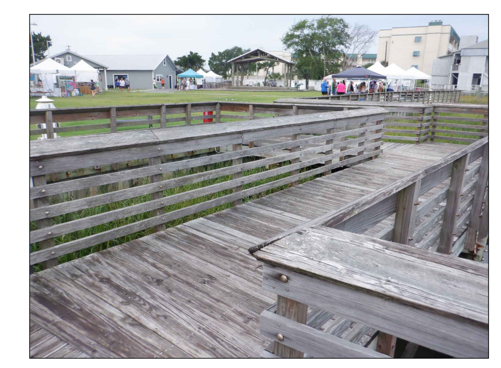
PHOTOGRAPH 2 - OVERVIEW LOOKING SOUTH
