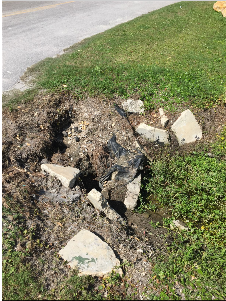
Clogged Culvert (Myrtle St.)
