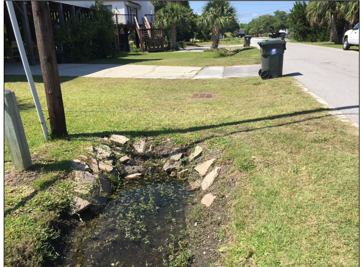
Standing Water along Billow St.
