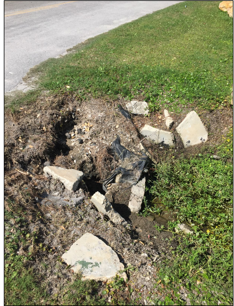
Clogged Culvert (Myrtle St.)
