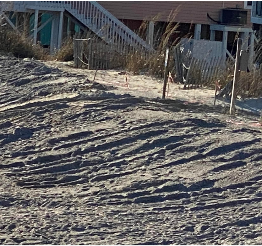
Repaired dune through sand scraping
