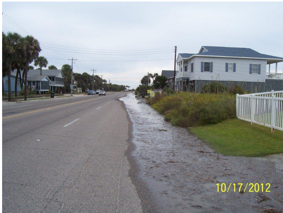
Figure 4.4: Recent photograph of high tide in Reach 15.
