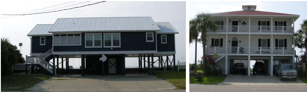
Figure 3.13: Examples of some typical structures along the Edisto Beach shoreline.
