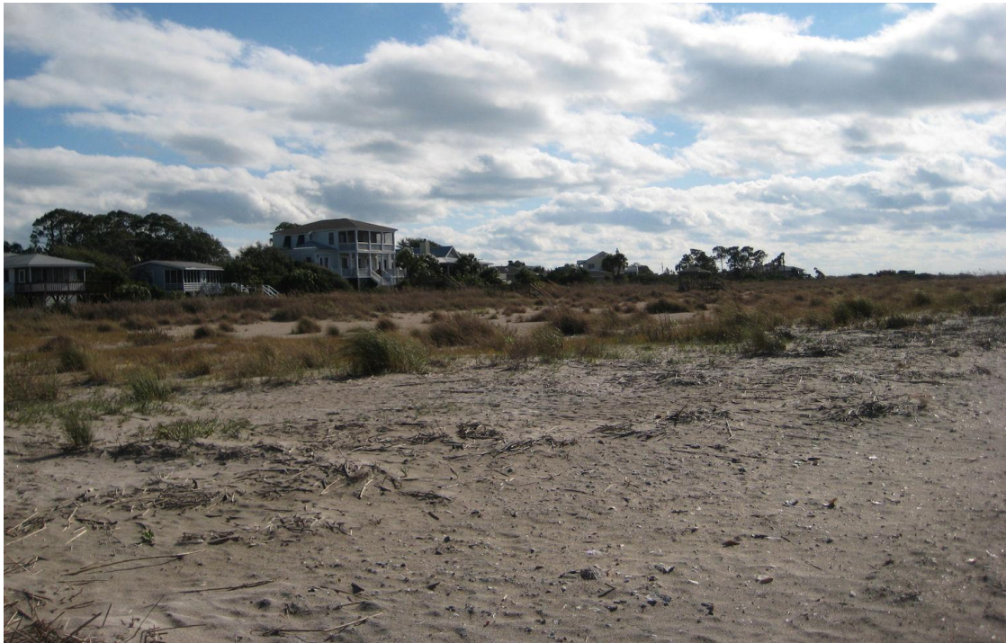
Figure 3.4: Example of a wider berm at the southern end of Edisto Beach. Photo dated November, 2011.
