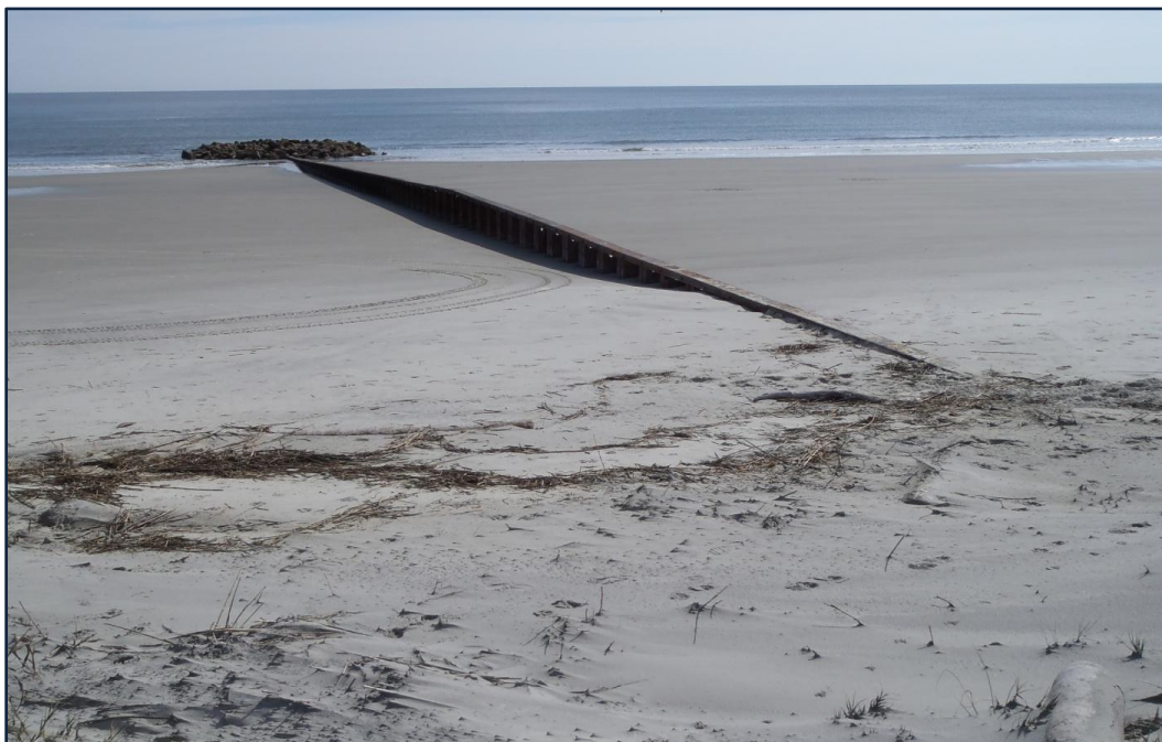
FIGURE 4. A Hunting Island (SC) groin built in 2007 showing the three recommended sections which are designed to follow the natural slope of the beach: upper dry beach section (berm), sloping wet-beach section (beach face), and low-tide section (low-tide terrace). Note the broad apron of loose armor stone at the head of the structure placed to reduce scour. This functions as a “T-head” and is considered to improve the performance of the groin.
