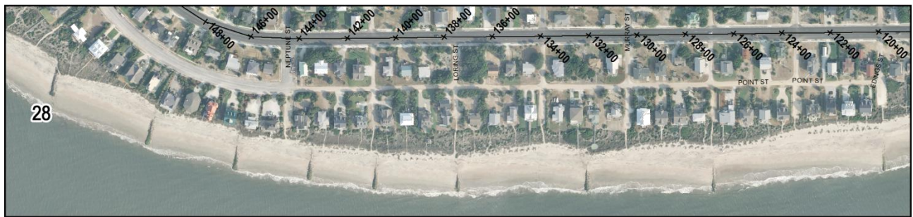
FIGURE 5. Reference baseline running along the centerline of Palmetto Boulevard. The baseline begins at Groin 1 (station 0+00) and extends to the southwest ~15,000 ft to Groin 28.
