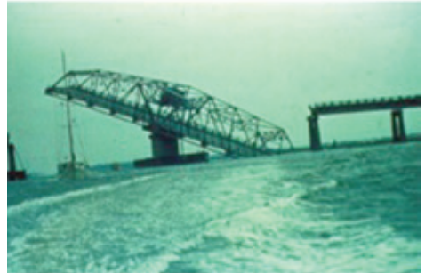
Figure 5. During Hurricane Hugo in 1989, (top) a new inlet formed on Pawleys Island; and (bottom) the Ben Sawyer Bridge collapsed, near Charleston, South Carolina. Photos courtesy of NOAA.
