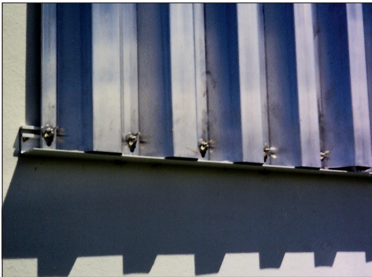
Figure 2. Metal panel shutter . The shutter is installed in a track permanently mounted above and below the window frame. The shutter is placed in the track and secured with wing nuts to studs mounted on the track. This type of shutter is effective and quickly installed, and the wing nut and stud system provides a secure anchoring method. Track designs that have permanently mounted studs for the nuts have been shown to be more reliable than track designs using studs that slide into the track.
