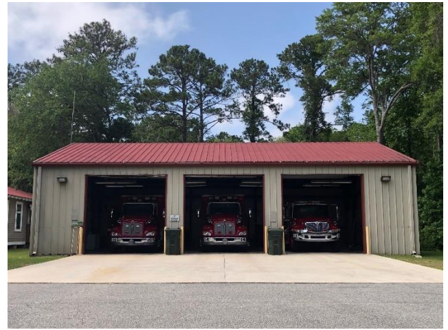
Photo by: LCOG—Colleton County Fire Station 20
