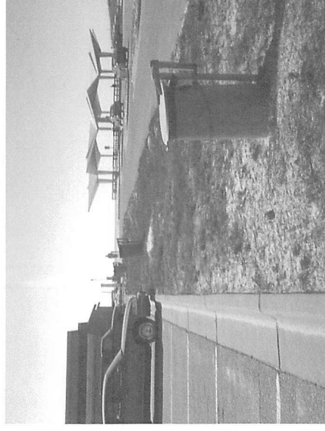
Example of trash receptacle anchored into the ground so it is not easily turned over.
