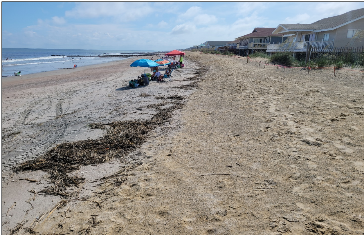
FIGURE 4.7. [UPPER] Cell 3 in July 2020 — the 2017 project was followed by sand fencing and vegetation plantings, which helped spur the initial stages of dune growth (seen on the right side of the frame). The wrack line located along the dune toe is evidence of high-water conditions reaching the dune ridge recently. [LOWER] Cell 3 in August 2021 — the darker-colored material on the right-hand side of the image is from the January-February 2021 dune restoration project, which used upland material to re-establish a protective storm berm and foredune. [Photos by D Giles]
