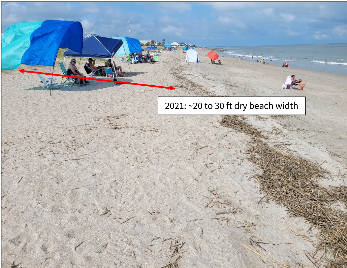
FIGURE 4.11. [UPPER] Cell 20 looking north in August 2015, before nourishment. [LOWER] Cell 20 looking north in July 2021. Although the dune is not fully visible in the lower photograph, the relative positions of the wrack line in each photo highlight the expansion in dry beach area since project completion. [Photos by D Giles]
