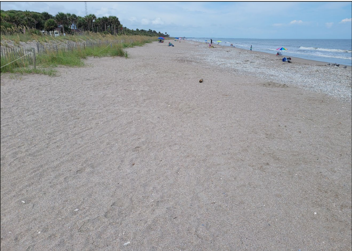
FIGURE 4.4. [UPPER] Upcoast 1 in July 2021. This reach has accreted since nourishment in 2006, transitioning from a washover barrier to a stable beach with a growing dune ridge. [LOWER] Upcoast 2, taken from just north of the Pavilion in July 2021.
