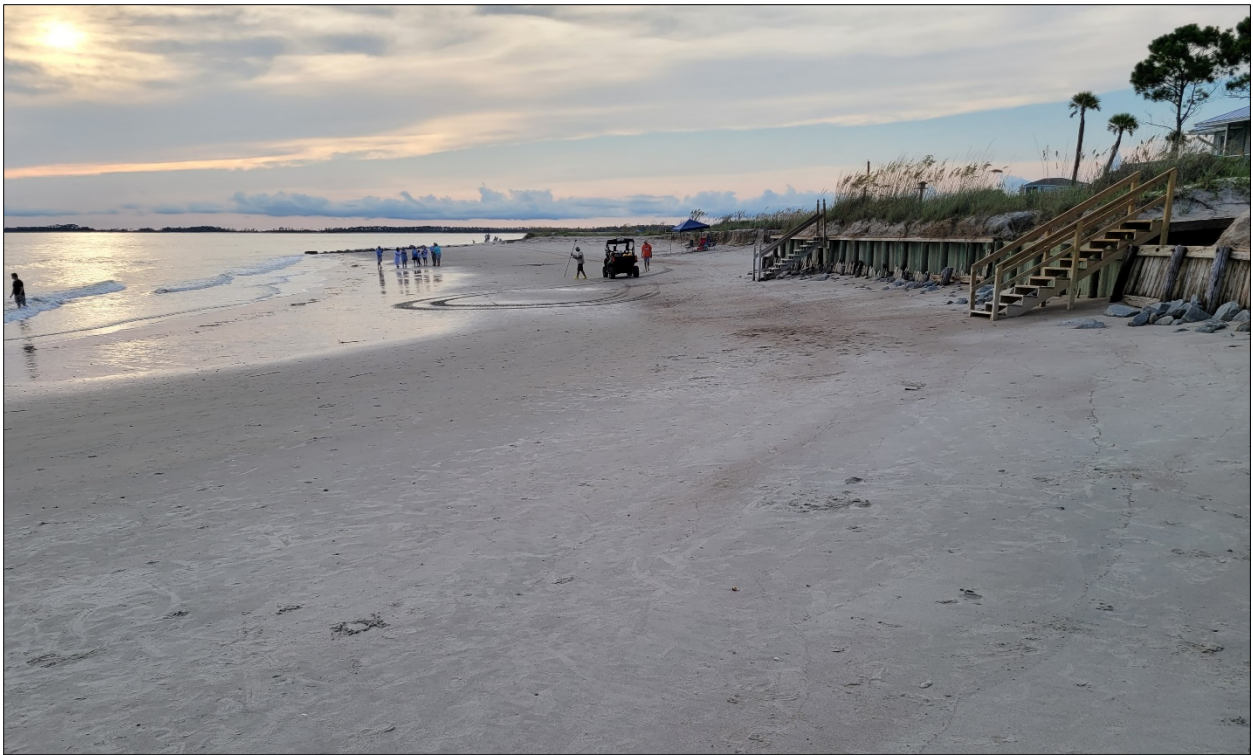
FIGURE 4.17. [UPPER] View west from Groin 29 in July 2020. [LOWER] The same area in July 2021. The erosional arc extending inland on the downdrift side of Groin 31, is more pronounced this year such that a low timber revetment is now exposed to wave action at high water conditions. [Photos by D Giles]
