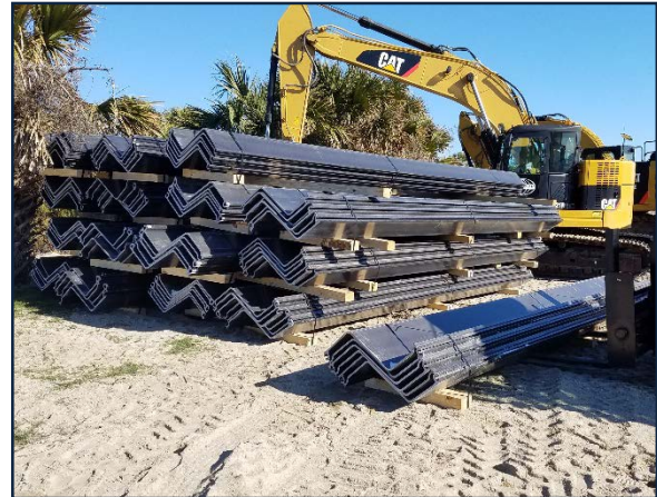
FIGURE 2.13. Staging of UC95 composite sheet piles.
