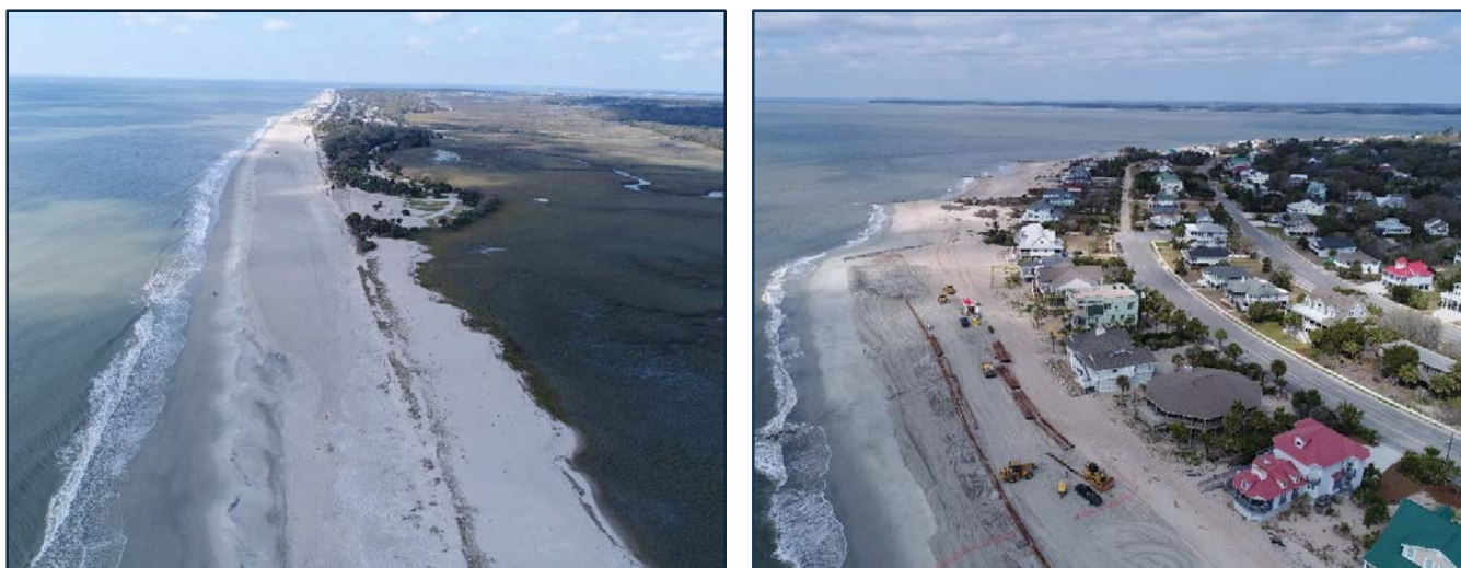
FIGURE 3.4. [LEFT] The completed beach at the state park. [RIGHT] Fill progress around Groin 27 at “The Point.”
