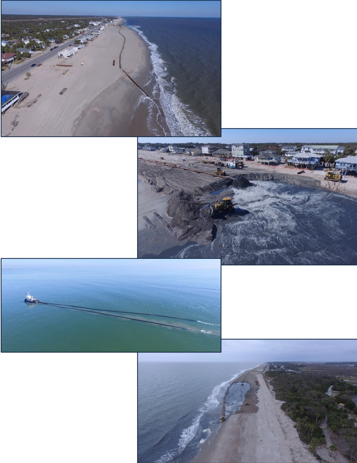
FIGURE 3.3. [UPPER LEFT] Early in the nourishment project, showing the subline coming onshore and the nourishment fill moving north. [CENTER RIGHT] The active fill area showing slurry coming from the discharge pipe. [CENTER LEFT] A tug towing new 500-ft sections of plastic shore pipe to the beach. [LOWER RIGHT] Fill in the state park area.
