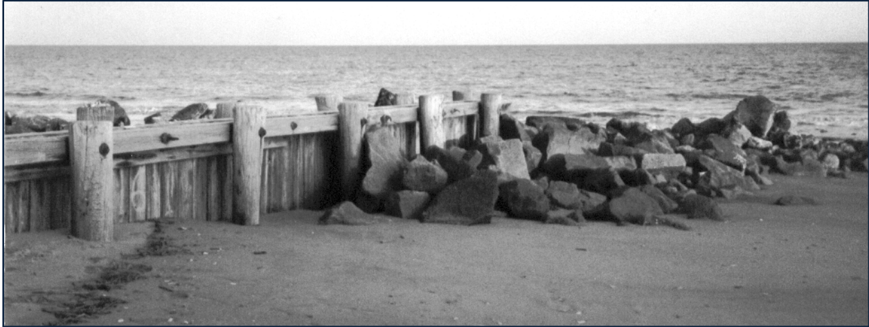
FIGURE 2.4. Typical Edisto Beach (SC) groin prior to the 1995 repair project.
