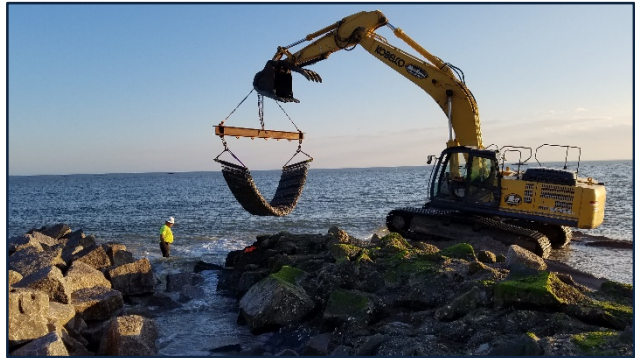
FIGURE 3.7 Images of the groin construction.
