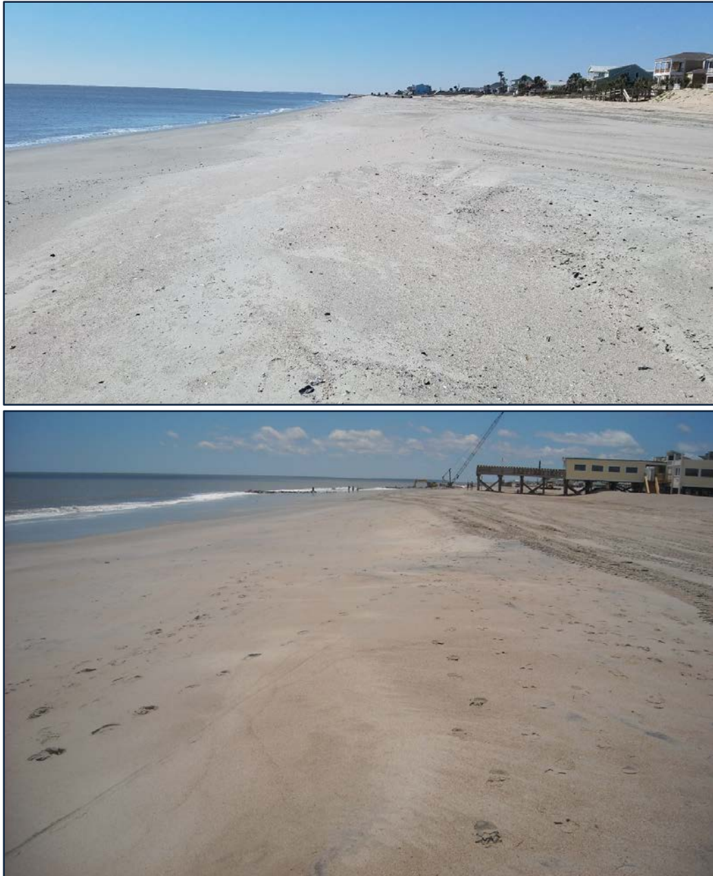
FIGURE 5.1. Example of sediment character of the fill sand. As the dredge moved within the borrow area, sediment characteristics changed slightly. Over time, exposed sediment will become more uniform over the length of the beach.
