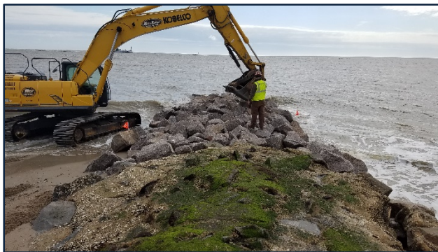
FIGURE 3.7 Images of the groin construction.
