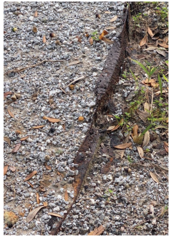
RUSTED PATH EDGING
